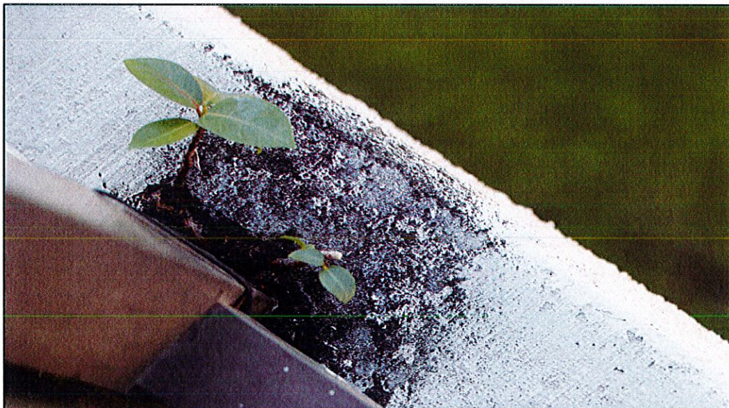
Photo #2. View of post base deteriorated grout and visible vegetation growth (unit 306 balcony).
