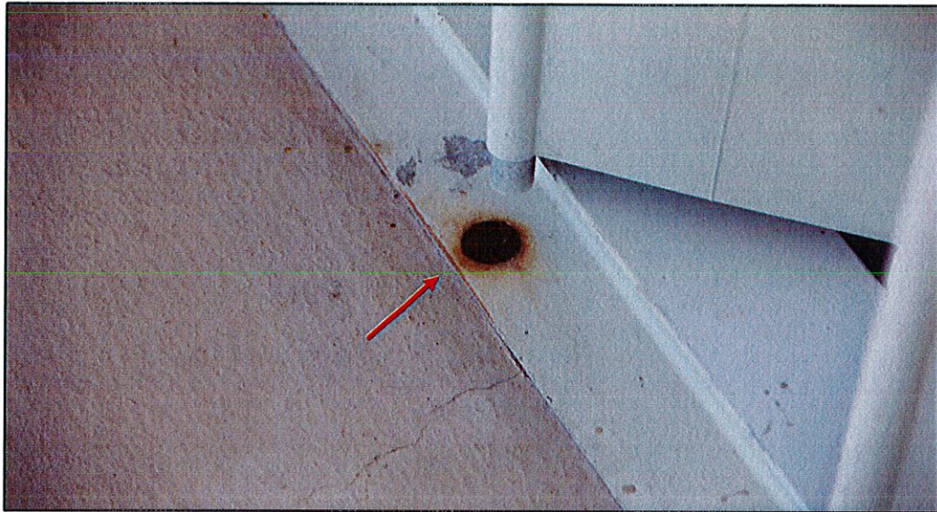
Photo #9. View of deteriorated metal anchors for the hurricane shutters. Observed at several units (unit 406 shown).
