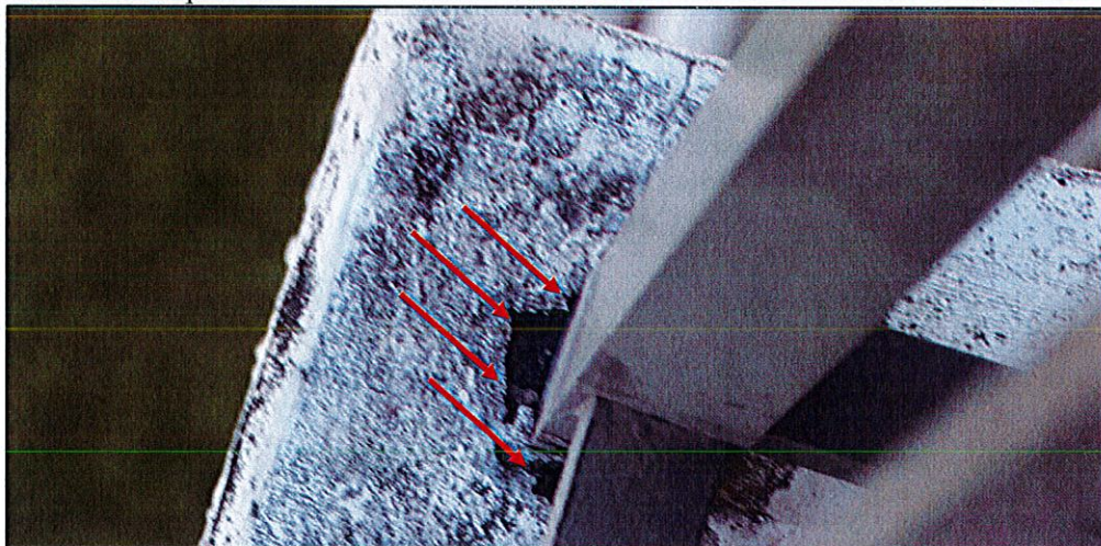
Photo #4. View of post base deteriorated grout with large gaps and metal post with signs of corrosion damage (unit 404 balcony).
