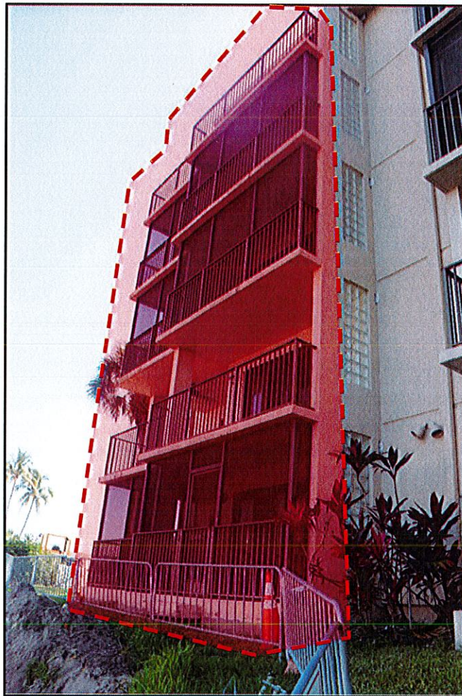
Photo #1. Building 1301 - View of line 06 balcony area affected by the seawall repairs.
