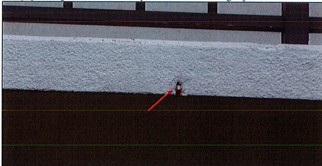
Photo #11. Close up view of embedded metals within concrete slabs with visible corrosion stains (unit 204 front corridor).
