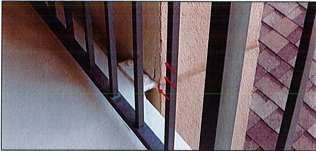
Photo #5. View of deteriorated stucco finishes at wall in front of stairs, signs of concrete spalling due to corroded reinforcing, condition observed at wall in front of elevator next to unit 303 front corridor.
