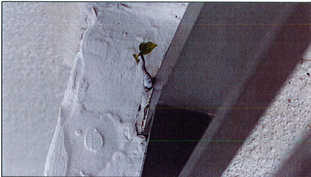
Photo #2. View of post base deteriorated grout and visible vegetation growth (unit 506 balcony).
