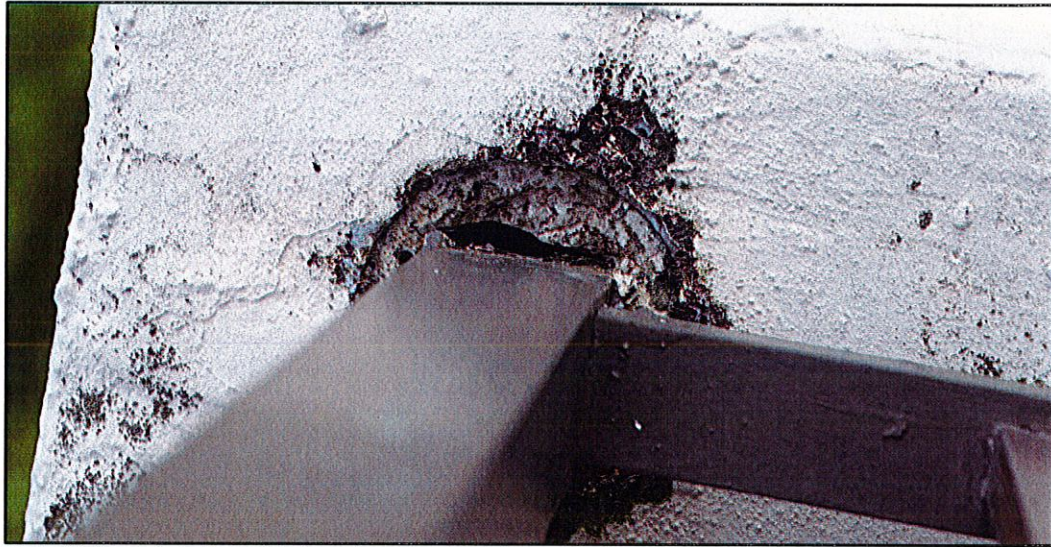
Photo #1. View of post base deteriorated grout and metal post with signs of corrosion damage (unit 506 balcony).
