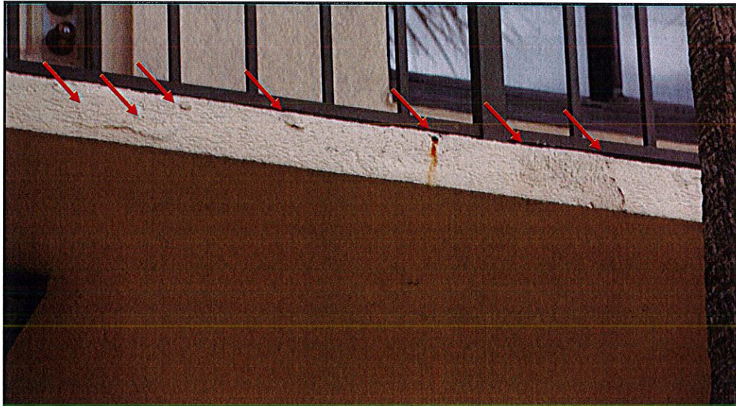
Photo #8. View of exterior stucco finishes with localized bulging and embedded metals with corrosion stains (unit 301 front corridor).
