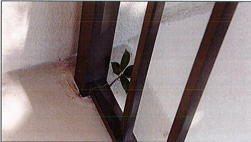
Photo #2. View of post base deteriorated grout and visible vegetation growth (unit 206 corridor).
