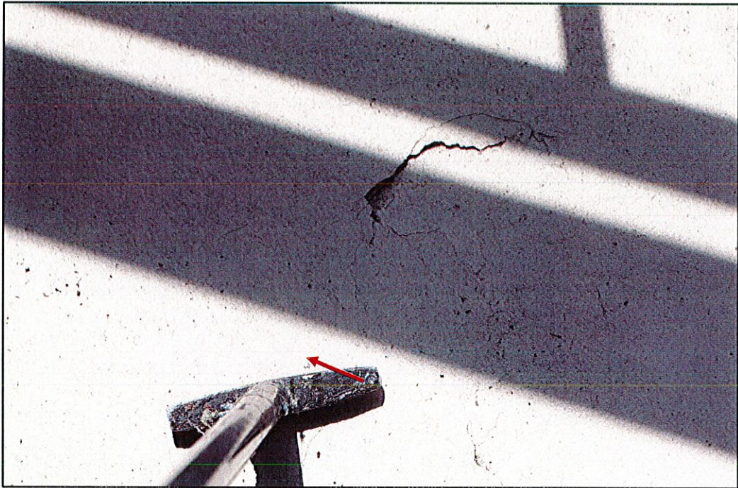
Photo #6. View of deteriorated floor finishes, signs of concrete slab spalling due to corroded reinforcing, condition observed at floor (Top of slab) of unit 304 balcony.
