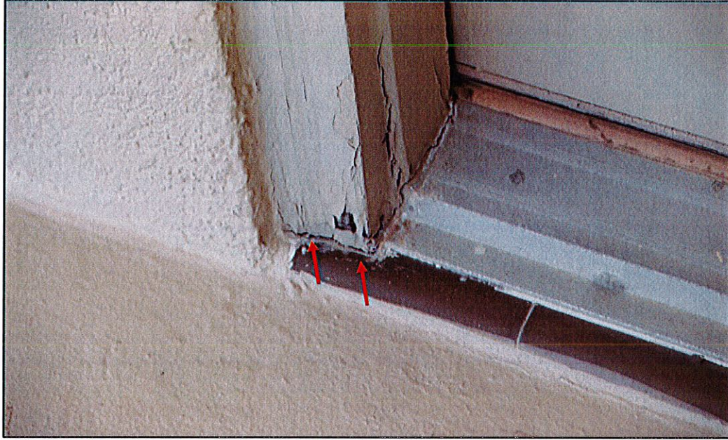
Photo #7. View of deteriorated sealant around the front door of unit 503.
