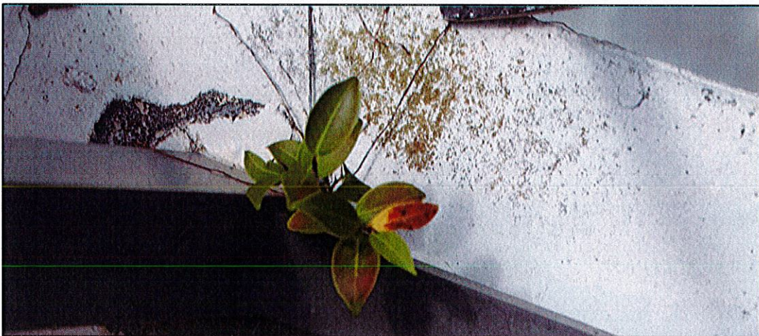
Photo #2. View of post base deteriorated grout and signs of organic growth (unit 406 balcony).
