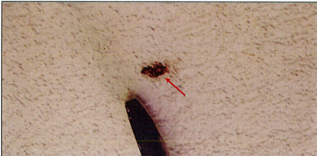
Photo #9. Close up view of embedded metals within concrete slabs. (Unit 402 balcony shown).
