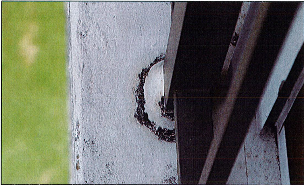
Photo #1. View of post base deteriorated grout and metal post with signs of corrosion damage (unit 502 balcony).
