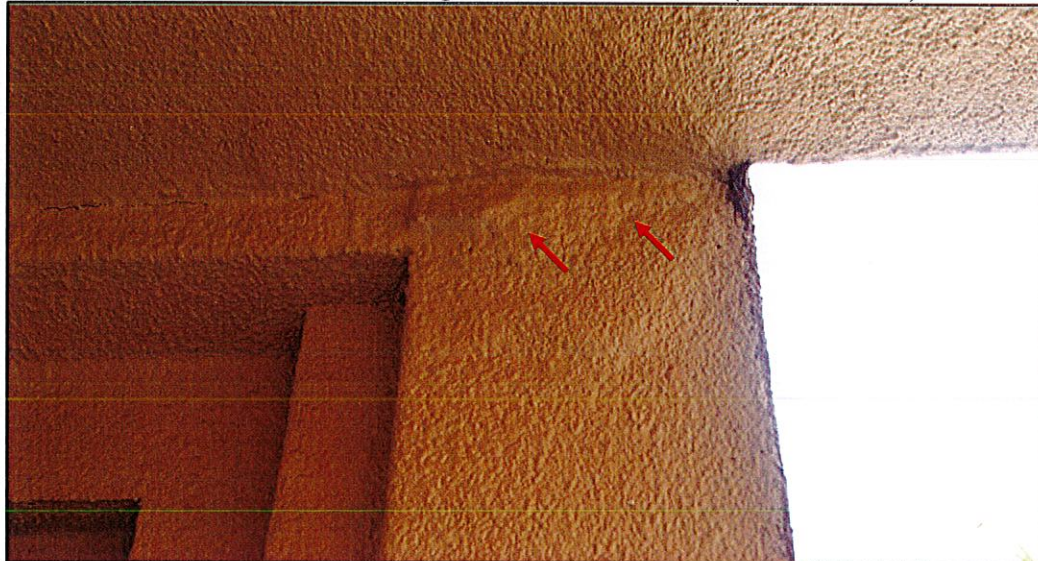
Photo #4. View of deteriorated ceiling stucco finishes, signs of concrete slab spalling due to corroded reinforcing, condition observed at ceiling of unit 305 front corridor.
