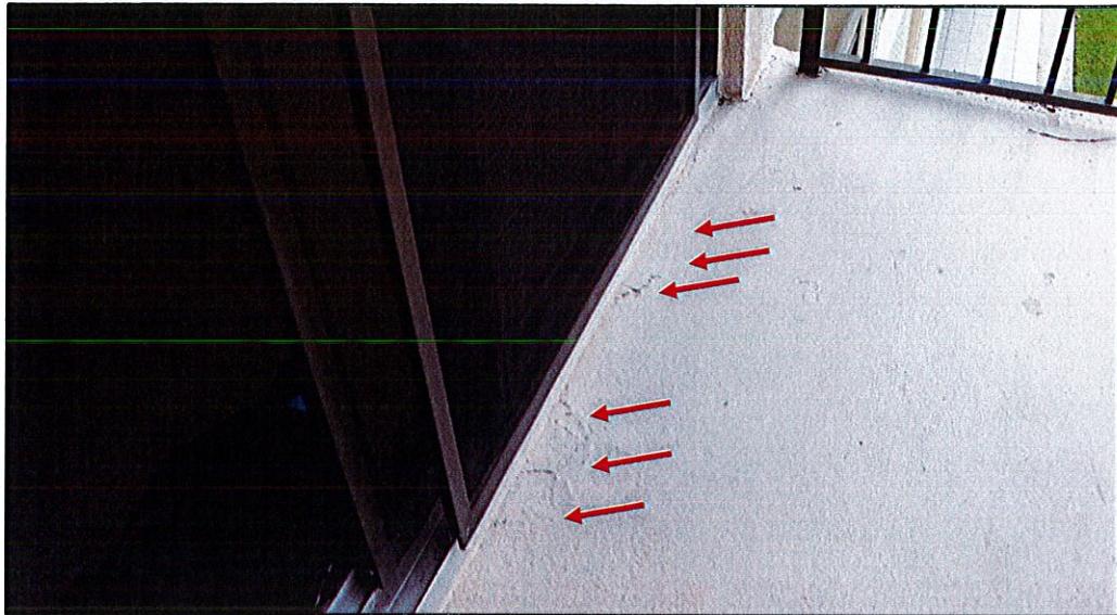
Photo #10. View of deteriorated floor finishes, signs of concrete slab spalling due to corroded reinforcing, condition observed at floor (Top of slab) of unit 305 balcony.
