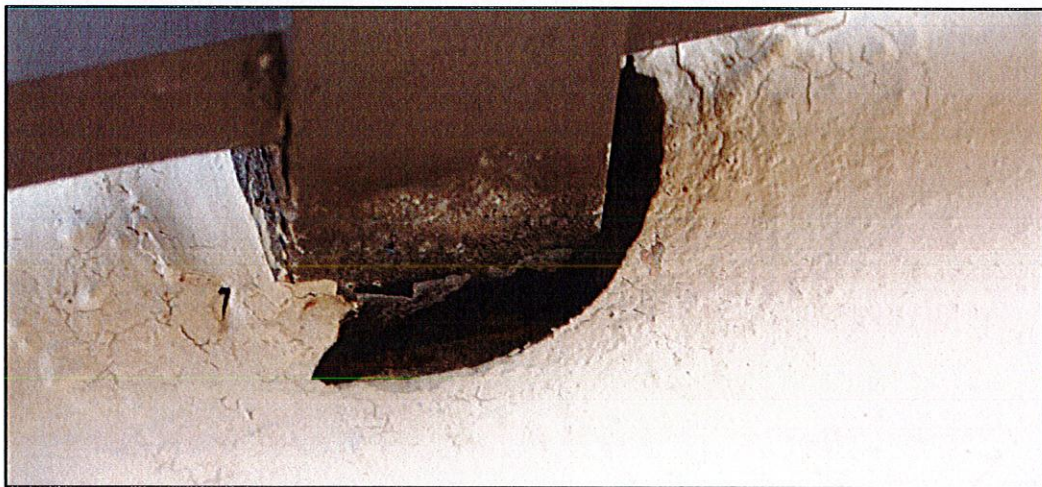
Photo #2. View of post base deteriorated grout and metal post with signs of corrosion damage (unit 402 front corridor).
