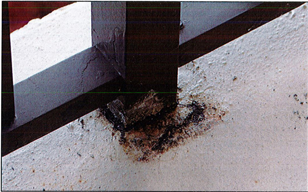
Photo #3. View of post base deteriorated grout and signs of organic growth (unit 202 front corridor).
