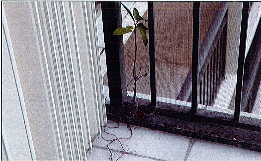
Photo #4. View of post base deteriorated grout and vegetation growth (unit 405 rear balcony).
