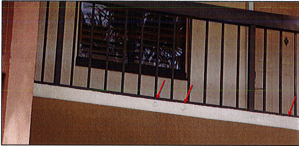
Photo #8. View of exterior stucco finishes with localized bulging (Ceiling of unit 206 front corridor).
