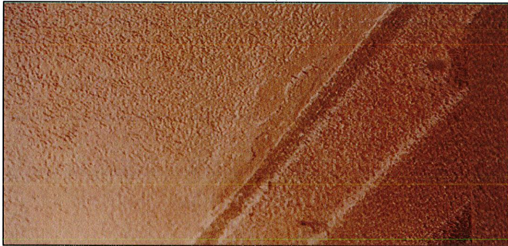
Photo #7. View of deteriorated ceiling stucco finishes, signs of concrete slab spalling due to corroded reinforcing, condition observed at ceiling in front of stairs between units 105 and 106.
