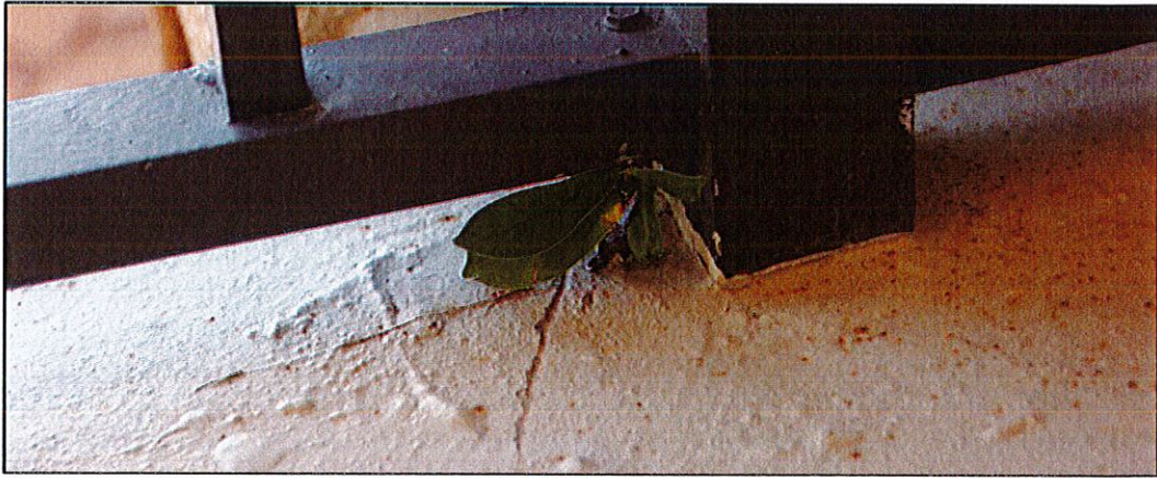
Photo #3. View of post base with vegetation growth (unit 304 front corridor).
