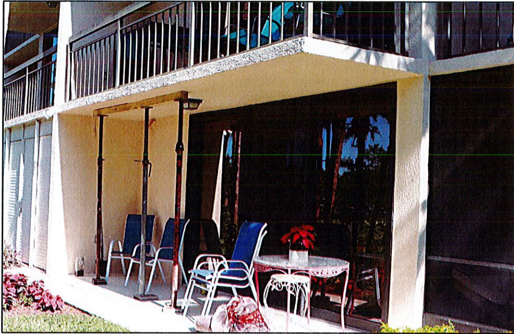
Photo #1. View of temporary post shores at balcony of unit 201.
