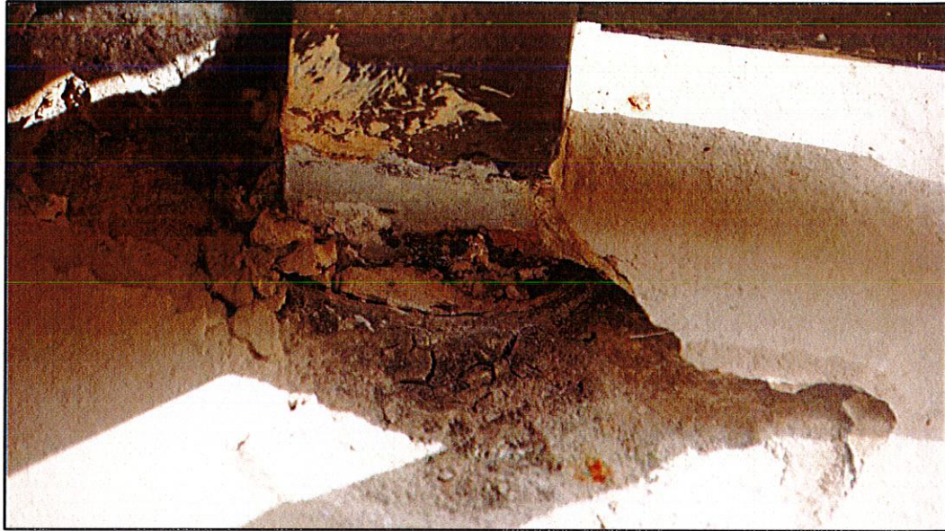
Photo #3. View of post base deteriorated grout and signs of organic growth (unit 203 front corridor).
