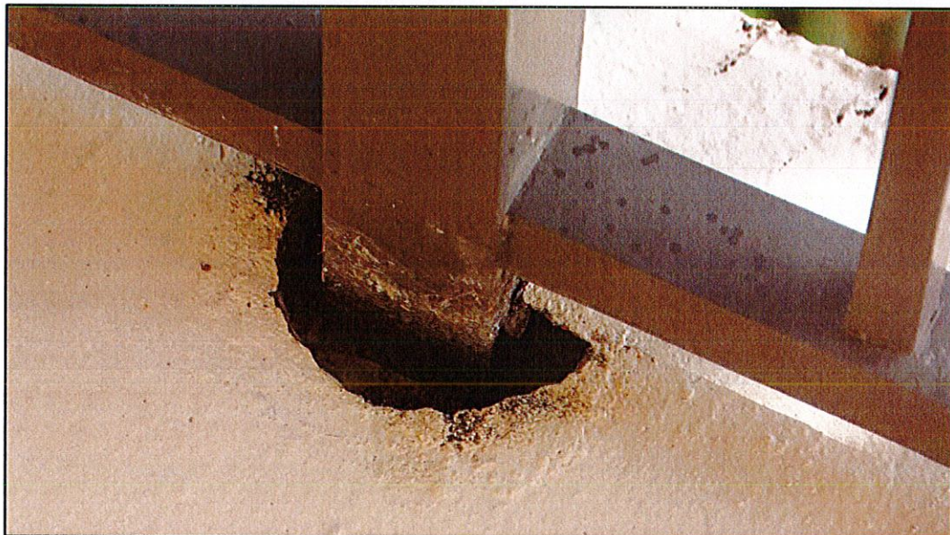
Photo #2. View of post base deteriorated grout and metal post with signs of corrosion damage (unit 305 front corridor).
