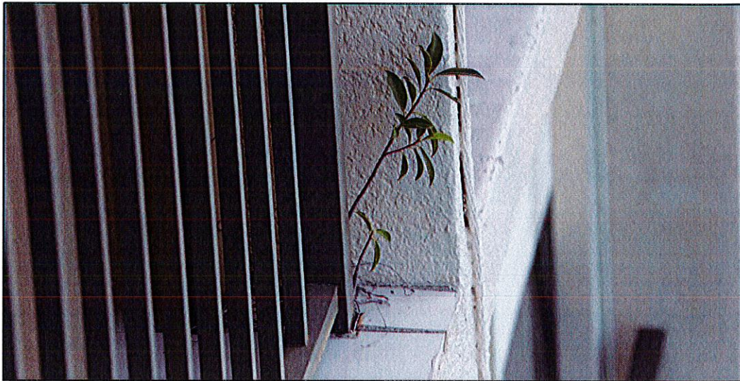
Photo #4. View of post base deteriorated grout and vegetation growth (unit 503 rear balcony).
