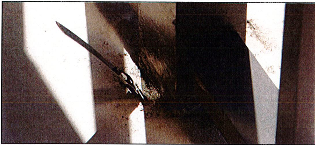
Photo #1. View of post base deteriorated grout and metal post with signs of corrosion damage (unit 404 front corridor).
