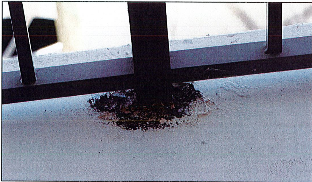
Photo #2. View of post base deteriorated grout and metal post with signs of corrosion damage (unit 402 balcony).
