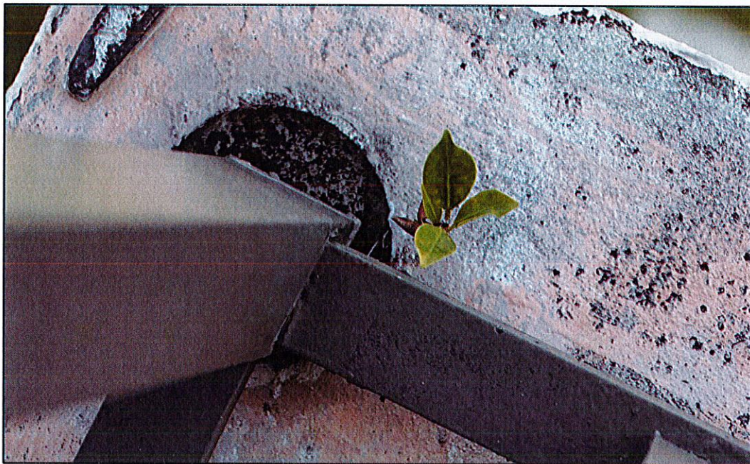
Photo #4. View of post base deteriorated grout and vegetation growth (unit 503 rear balcony).
