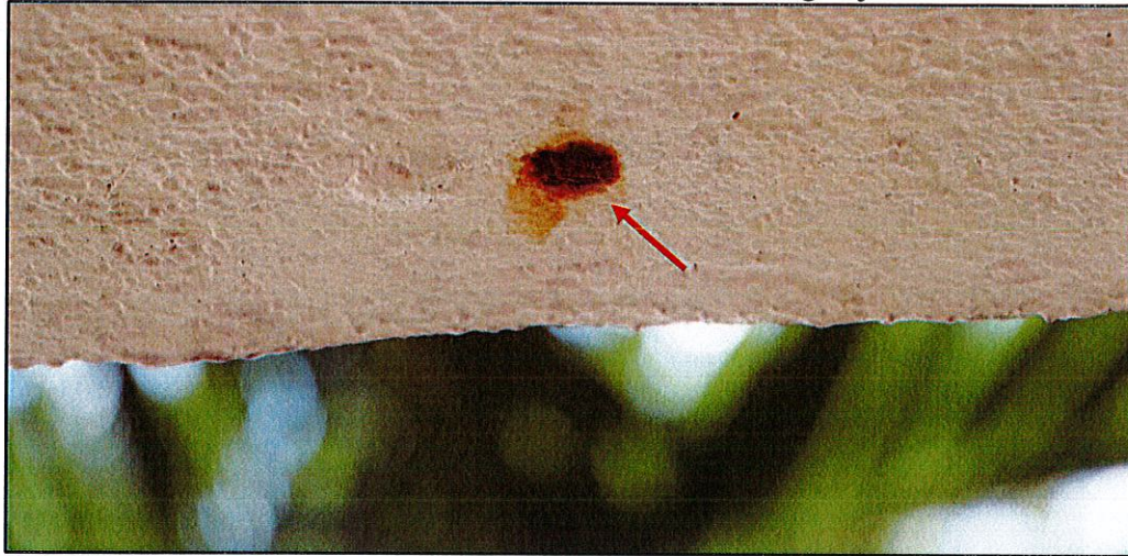
Photo #15. Close up view of embedded metals within concrete slabs. (Unit 104 ceiling balcony shown).
