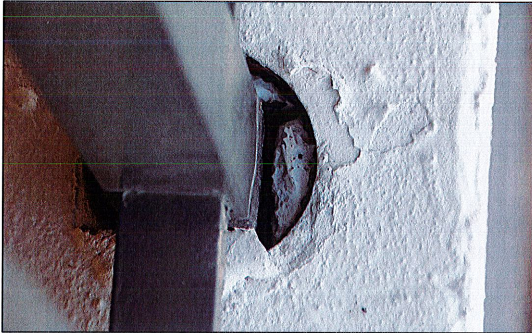
Photo #3. View of post base deteriorated grout and signs of organic growth (unit 505 balcony).
