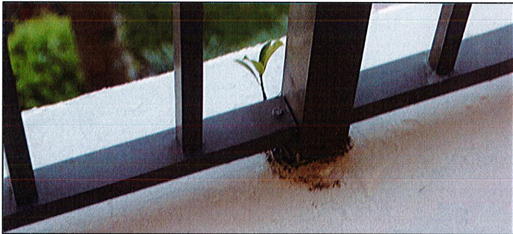
Photo #4. View of post base deteriorated grout and vegetation growth (unit 405 front corridor).
