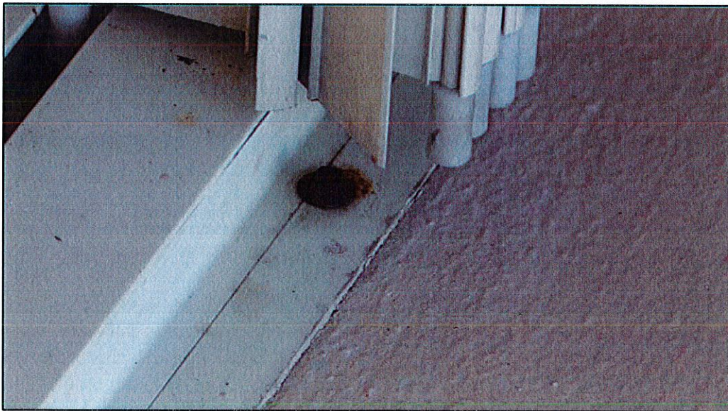
Photo #14. Close up view of deteriorated metal anchors for the hurricane shutters. (Unit 403 shown).
