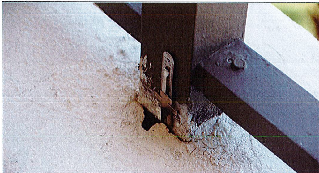
Photo #2. View of post base deteriorated grout and metal post with signs of corrosion damage (unit 402 front corridor).
