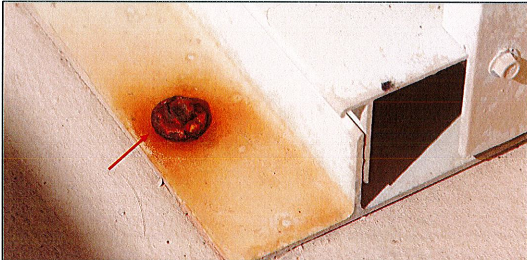
Photo #8. View of deteriorated metal anchors for the hurricane shutters. Observed at several units (unit 204 shown).
